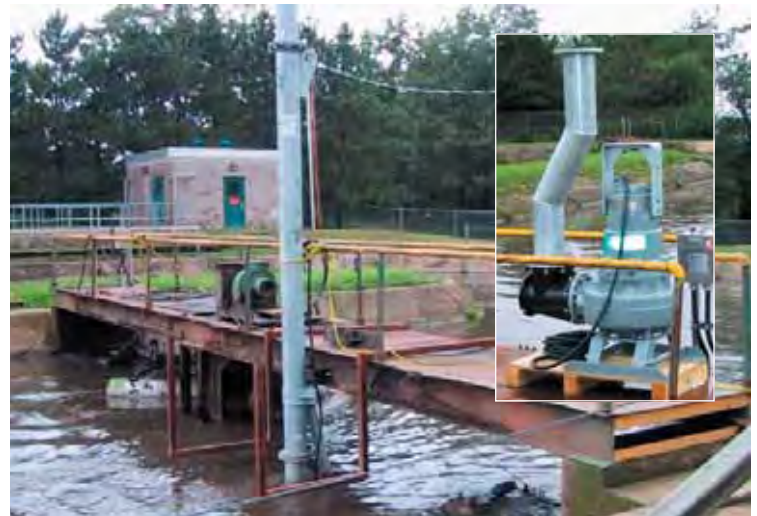
The complete Flojet Aeration System from Flygt. Shown in inset: the NS 3152 MT pump with a 117-150 ejector kit.
