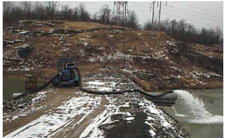
The Thompson 6-inch Compressor-Assisted Dry-Prime pump recirculated the acidic water and lime mixture to maintain pH levels.
