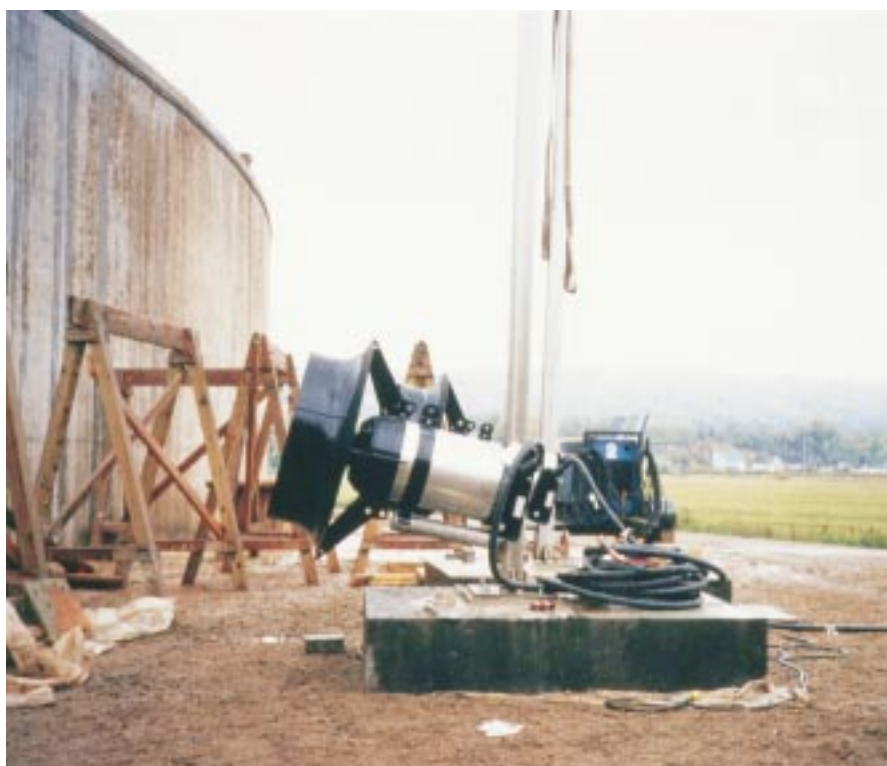
The mounting system of the SR 4680 submersible agitator allowed for installation without having to empty the basin.
