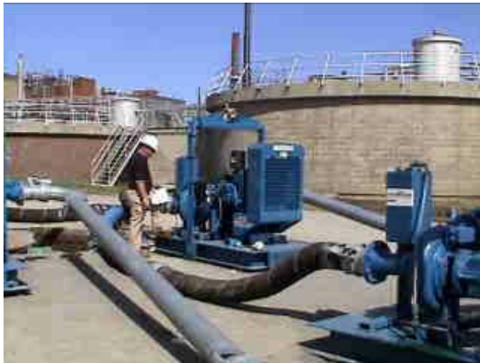
A worker supervising several Thompson diesel suction pumps on site.
