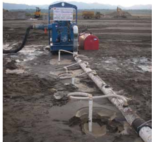
Diesel well point pump connected with header and swing pipes.
