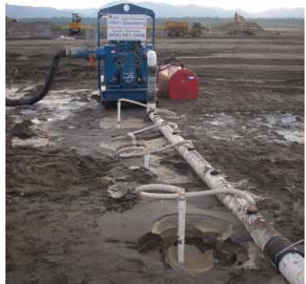
Diesel well point pump connected with header and swing pipes.
