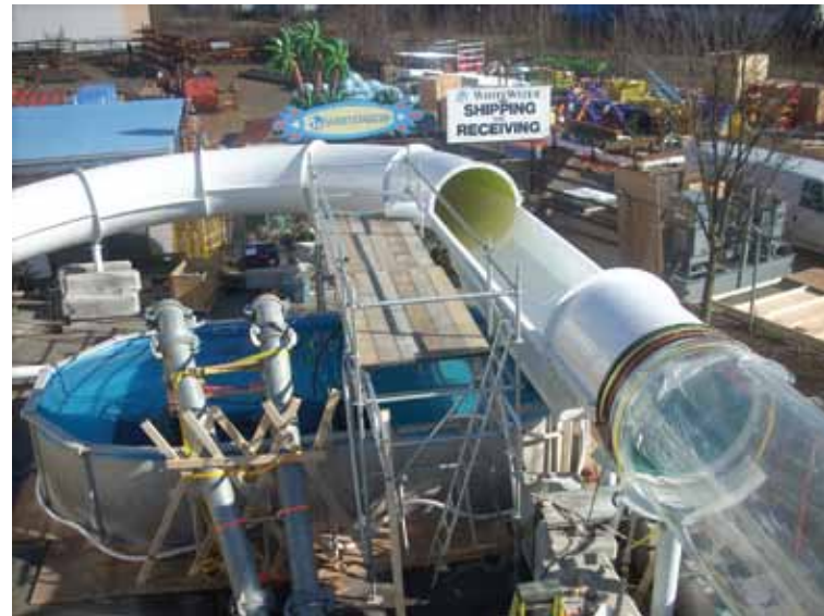
Aerial view of the test installation at Whitewater West Industries.
