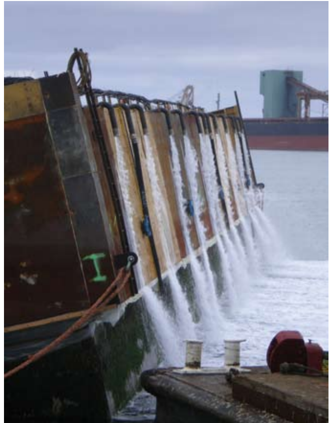
4" diameter special length hoses shown here evacuating the water from the top a caisson.
