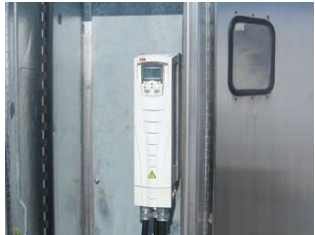
Flygt ACS550 Variable-frequency drive (VFD).
