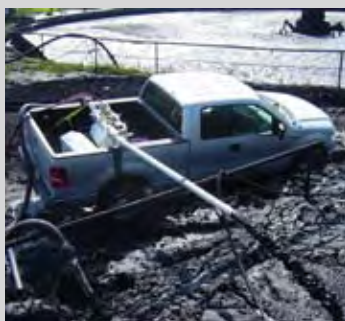
Mountains of settled coal easily transferred by SV60 on pickup.
