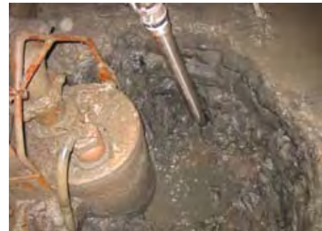
Guzzla SV60 in operation at 4130 level at CVRD Inco in Sudbury.
