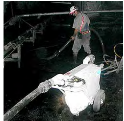
Guzzla SV60 mobile solids transfer pump cleaning up muck underground.
