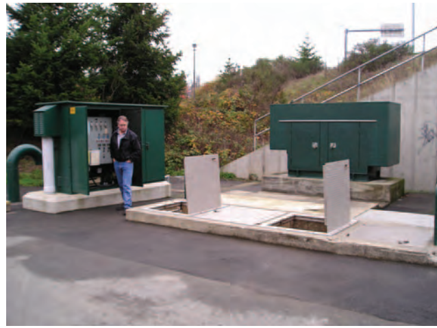
Emmett McCusker doing a regular station inspection.
