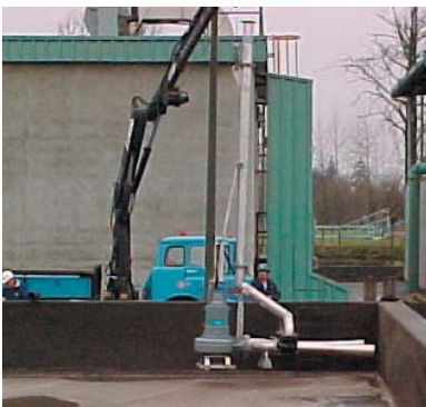
Units being lowered into the digester.
