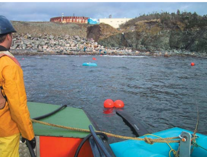
BS-2250 being tied off from the mooring lines approximately 100 feet from the low water level. The pump flotation module, model PFM 200, is used to keep the messenger off the bottom. The 150 kW generator and tank in question is in the background.
