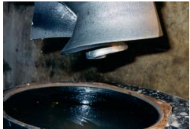
Clog-free impeller of the N-Pump after the three month trial period.
